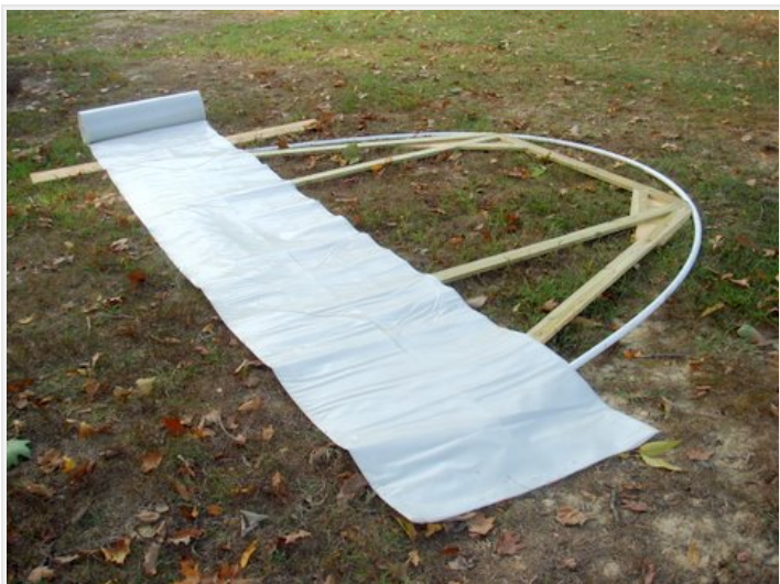
I just rolled the plastic out on the frame... Notice the falling leaves - I'm racing against fall weather with this project.
