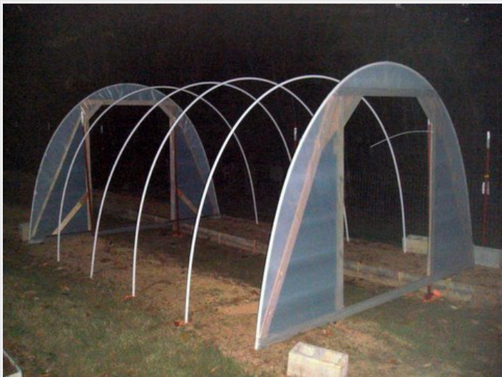
At this point it takes about 2 minutes to install the pvc pipes for the intermediate ribs - and the polytunnel takes shape. For a stronger, more permanent structure use more ribs and put them closer together - or even use larger pipe. I haven't tried it but I bet you could use up to 1 1/2" pipe - although you might have to bend it into shape on a warm day.
