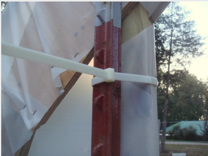
Tie the hoop house end frames to the fence posts with wire ties, wire or rope.
