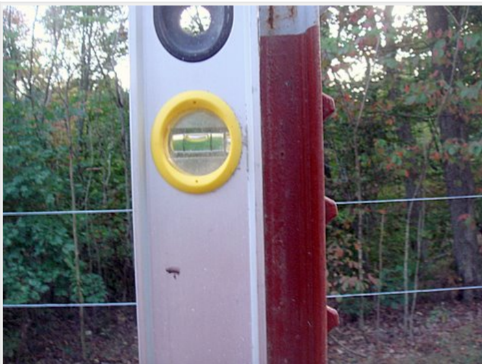
Check the fence posts for plumb and bend them a little if they need straightening.
