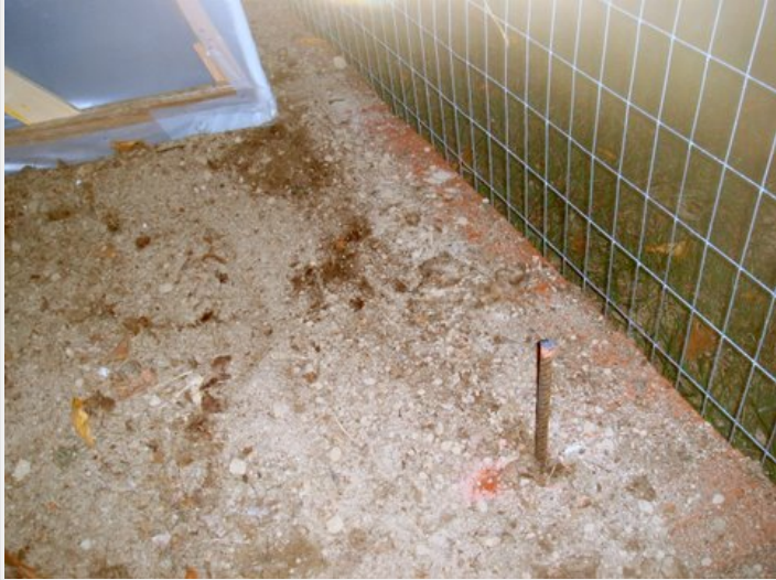
Drive rebar pins every 3 feet to secure the intermediate ribs...
